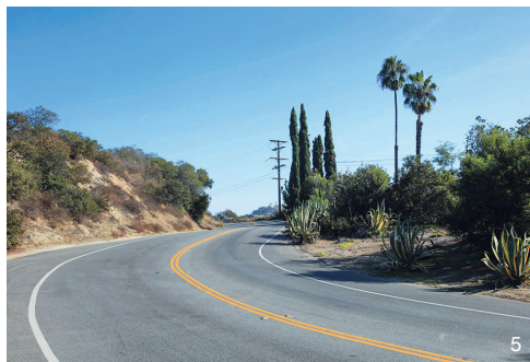
5 穆赫兰道已铺装段现状 Current conditions of the paved Mulholland Drive
